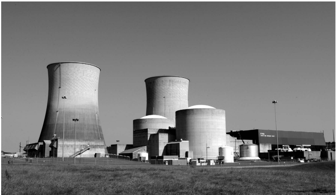
Figure 7. Watts Bar Nuclear-Generating Station
